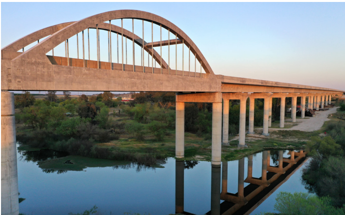
The San Joaquin River Viaduct is a signature structure and serves as the northern gateway into Fresno. This structure was completed in 2021.
