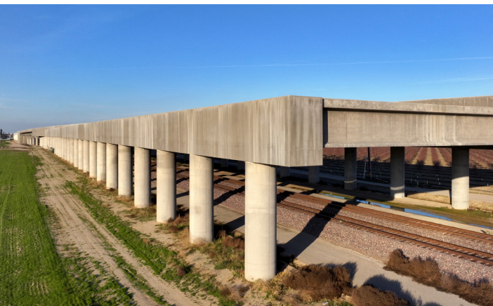
The Wasco Viaduct will take high-speed trains over the existing BNSF freight tracks and is nearly 2,000 feet long. It was completed in March 2023.
