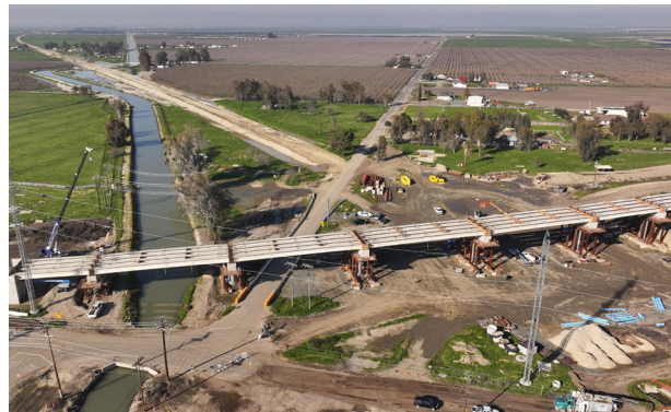
Corcoran Highway Grade Separation, Kings County, January 2026
