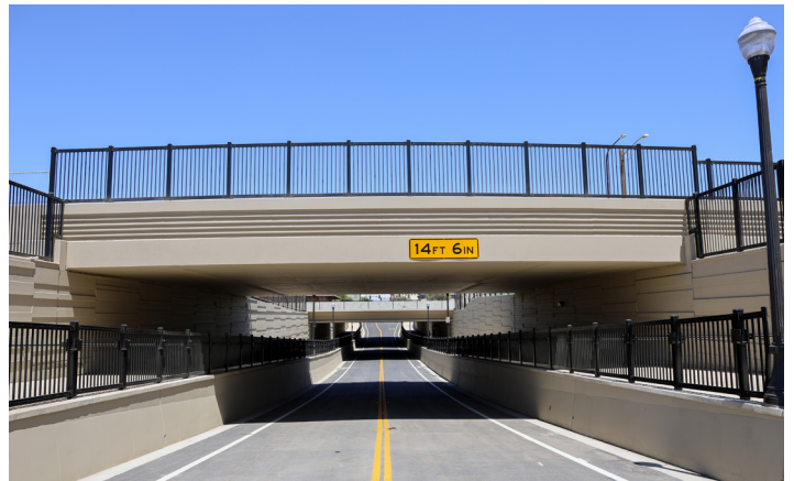
The Tulare Street Undercrossing was completed in July 2025 and takes traffic under the existing Union Pacific Railroad and future high-speed rail lines. This grade separation eliminated the previous grade crossing at Tulare Street.
